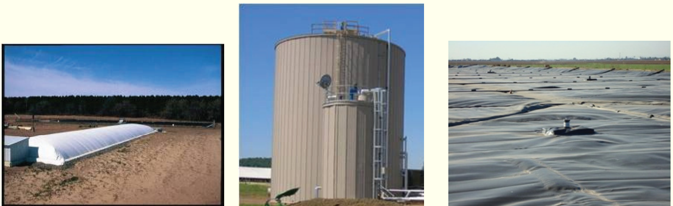
Figure 1. Plug-Flow Digester (left), Complete Mix Digester (center), and Covered Lagoon Digester.
